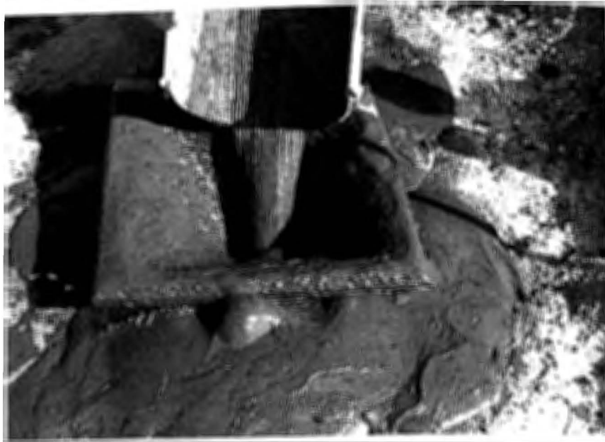
Flowable fly ash slurry is discharged from a ready-mix concrete truck into an abandoned steam utility manhole at Wisconsin Electric's Valley Power Plant in Milwaukee.
