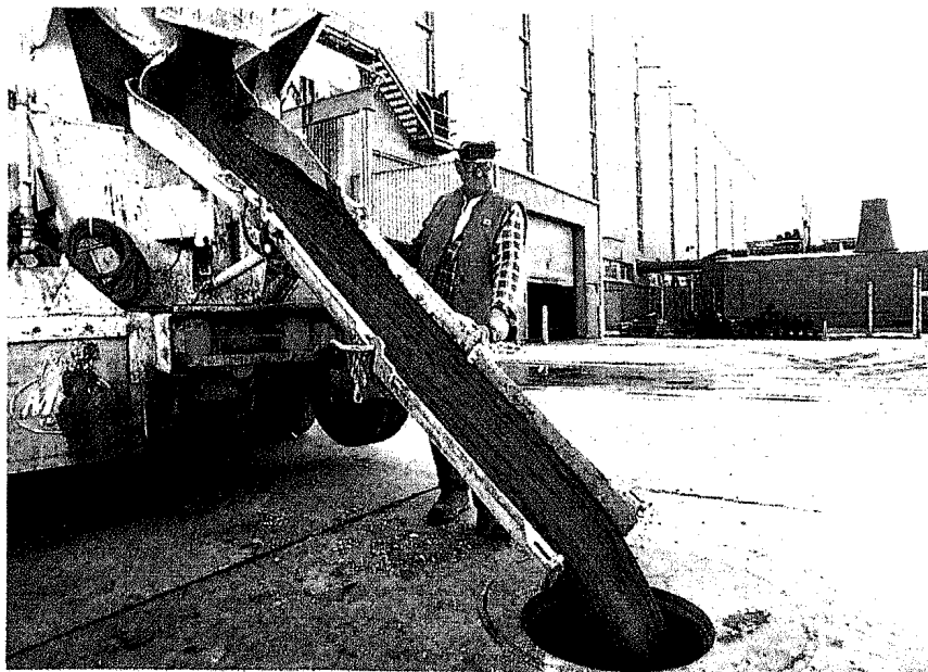
Flowable fly ash slurry is funneled into a 9½ ft diameter abandoned tunnel crossing the Menomonee River in downtown Milwaukee. The self-leveling material flowed over 235 ft.
