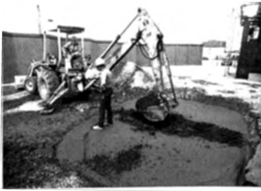
Because of its low strength, excavating the hardened CLSM is easily accomplished with ordinary excavation equipment.
