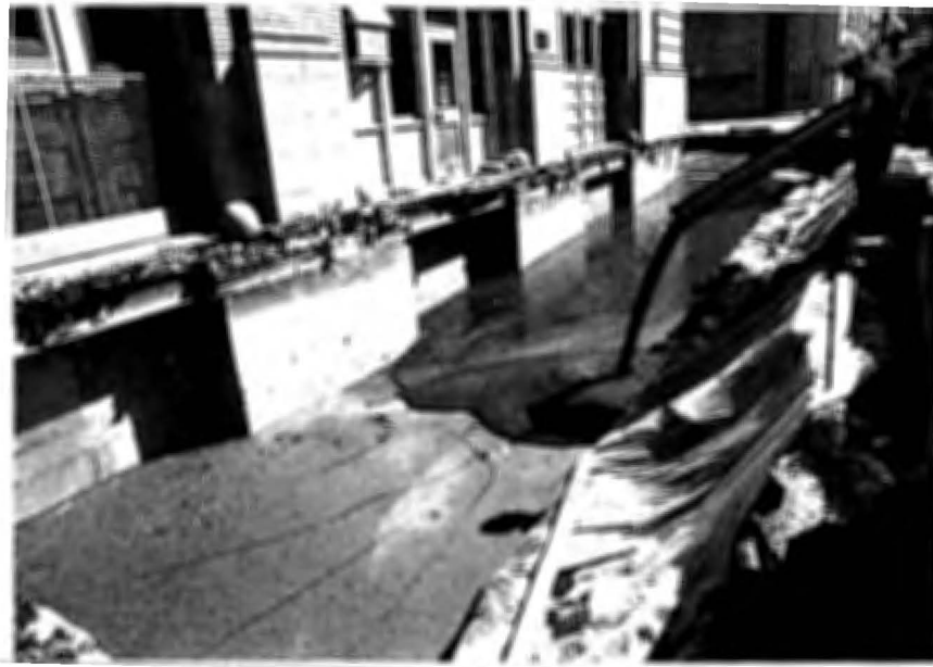
An abandoned sidewalk area was filled in lifts because of the high fluid pressure exerted on the basement wall.
